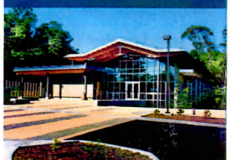
New Blue Ridge Parkway Visitor Center.
